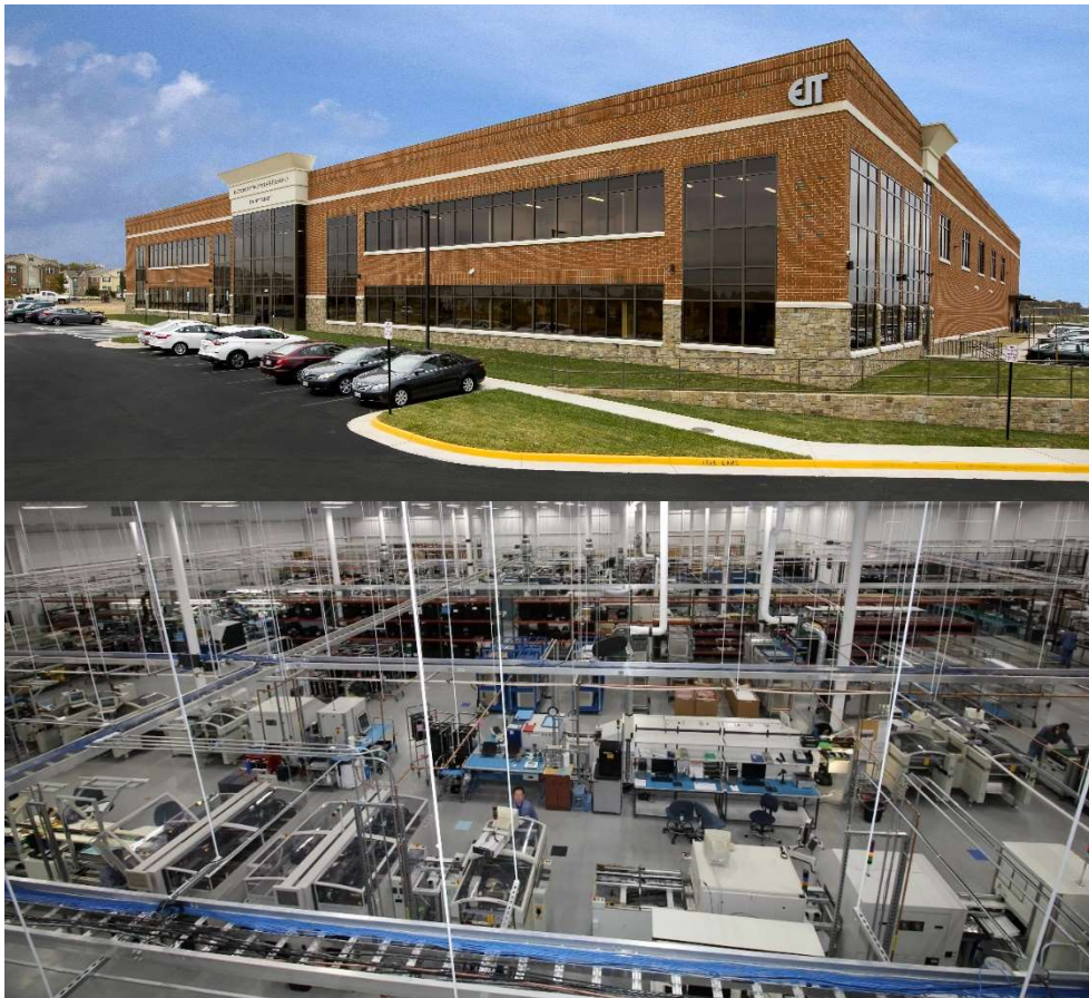
Figure 1: EIT Manufacturing Facility, Leesburg, VA
